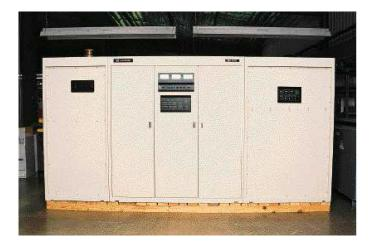
FIG.16 Harris 1 MW DX-LW Digital AM Transmitter
